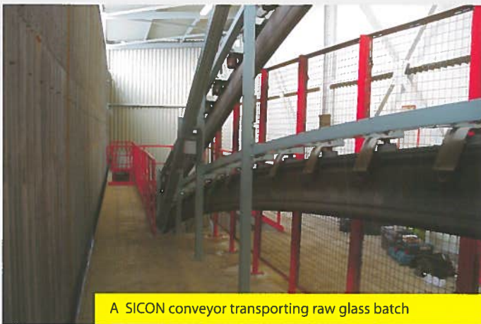
Limestone and gypsum handling systems
